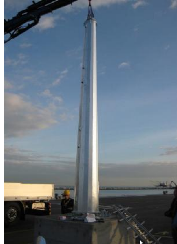
Small Wind Turbine erection
