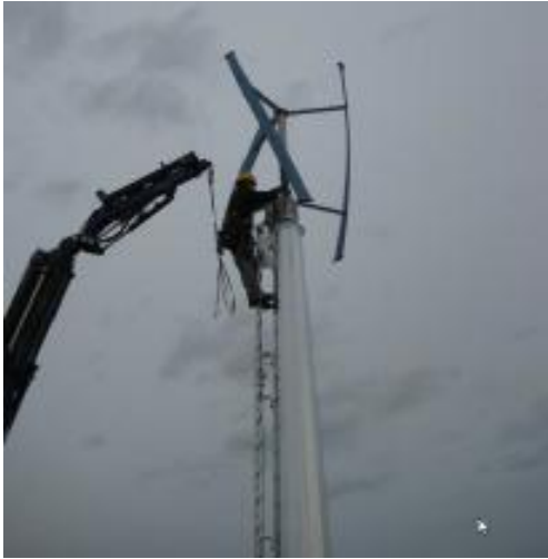
Small Wind Turbine mounting
